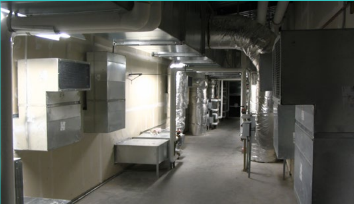
Wilson High School, NAC Architecture
